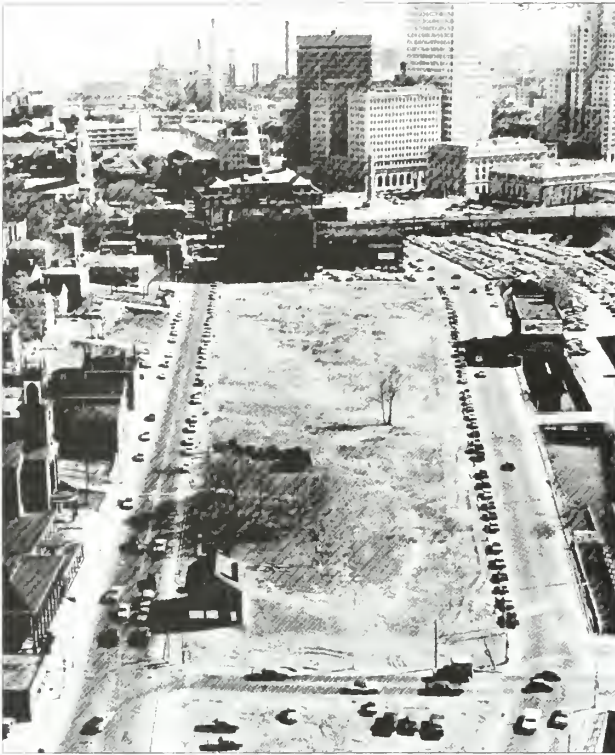
Figure 1.47. Looking south over the national memorial site in c.1975 following completion of demolition and site grading. The only remaining features on the site were the Antram-Gray House, which had been moved forty feet south of Smith Street (not widened until 1976), the Bernon Park grove, and Roger Williams Spring Park. (National Park Service, "Environmental Assessment of Development Concept Alternatives, Roger Williams National Memorial," February 1977.)
